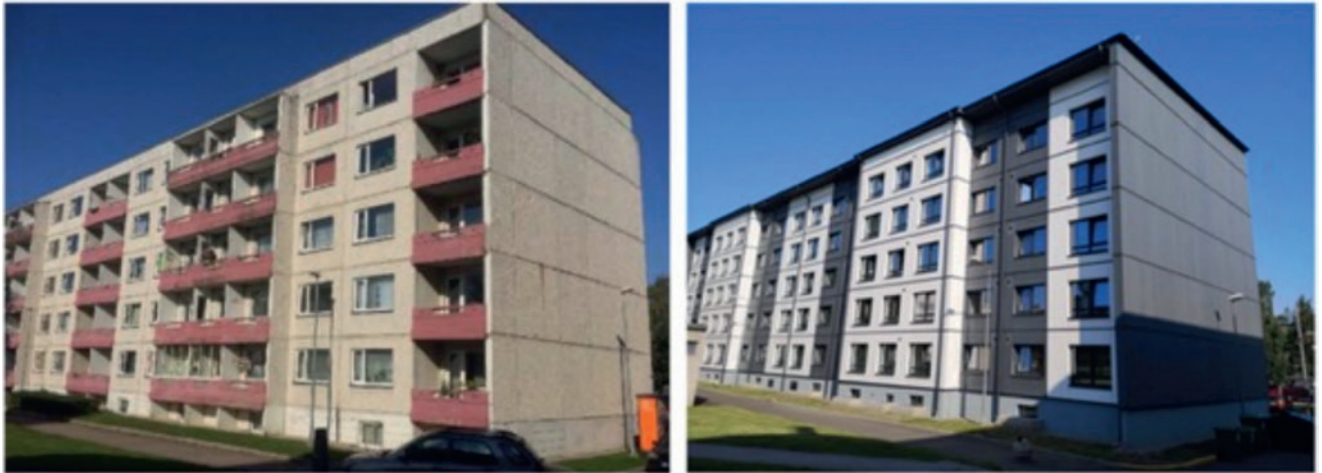
Figure 5 Apartment building in Estonia before refurbishment in 2015 (left) and after a low-energy refurbishment in 2018 (right) (source: Hamburg et al. 2020 ).
